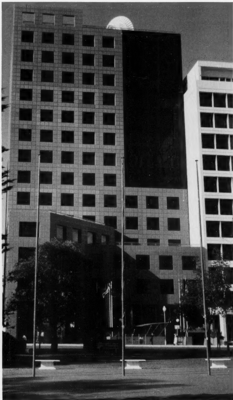
The consulate general occupies the top floor of this building, St. George's Court.
